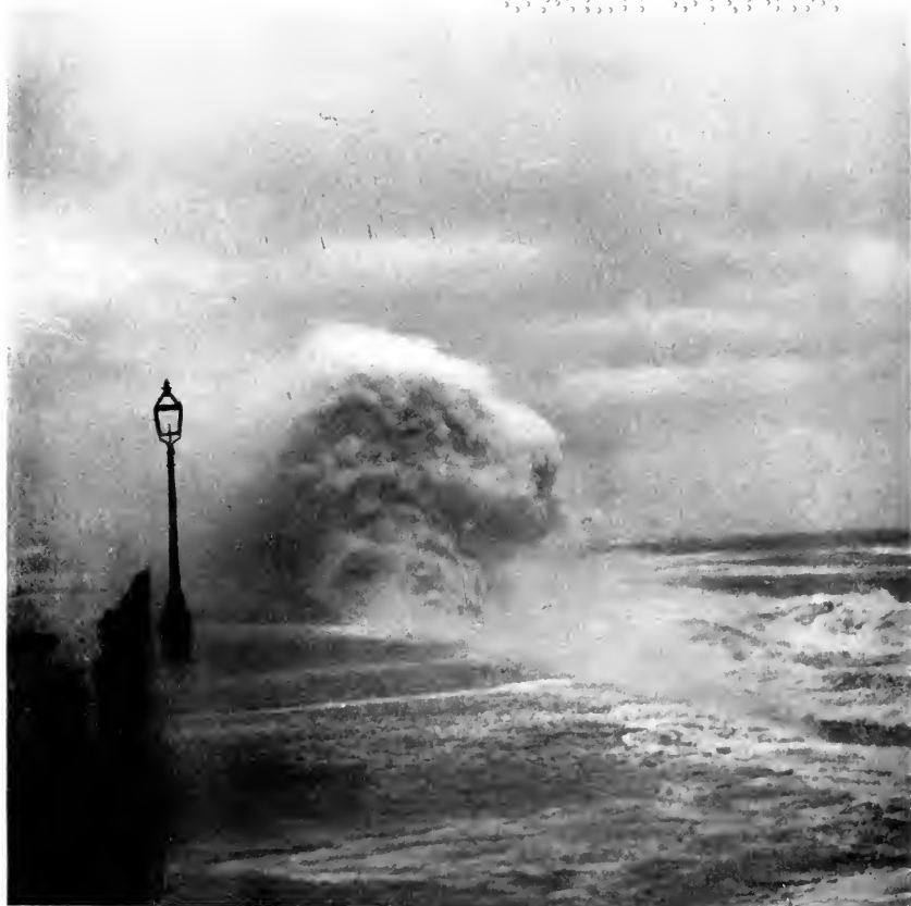
WAVE BURSTING AGAINST A VERTICAL WALL.
